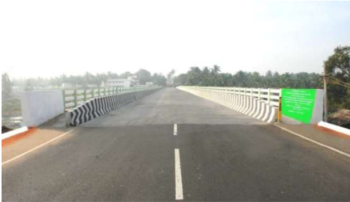
Hanumantheertham Bridge across Thenpennai River opened on 27.01.12 by the Hon'ble Chief Minister
