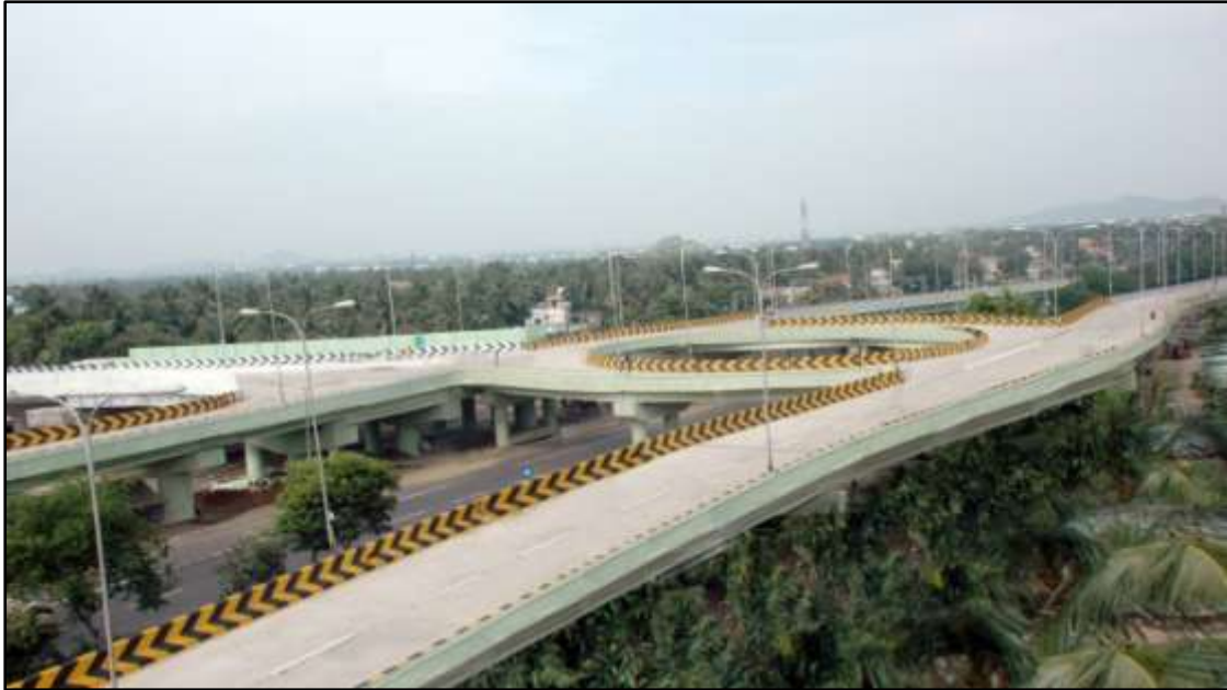
Vandalur Railway Over Bridge opened on 27.01.2012 by the Hon'ble Chief Minister
